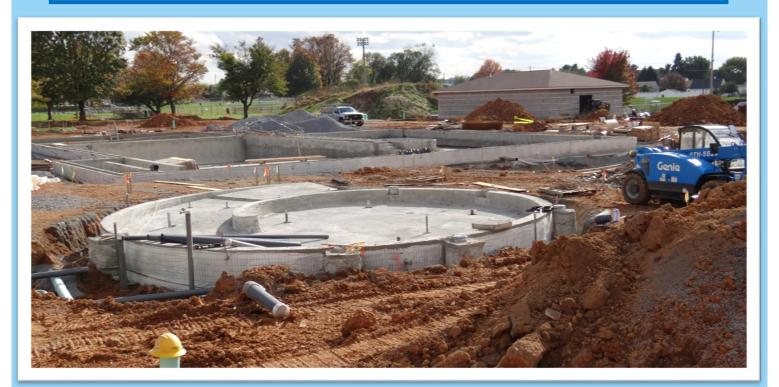
The two pictures below depict the skeleton of the Lazy River. The exterior walls will be sprayed, and then the final shotcrete process will be applied to the walls of the center island. Upon this completion, all pools will be ready for the final, applied finish and then filled! Get ready for a Splashtastic Summer!
